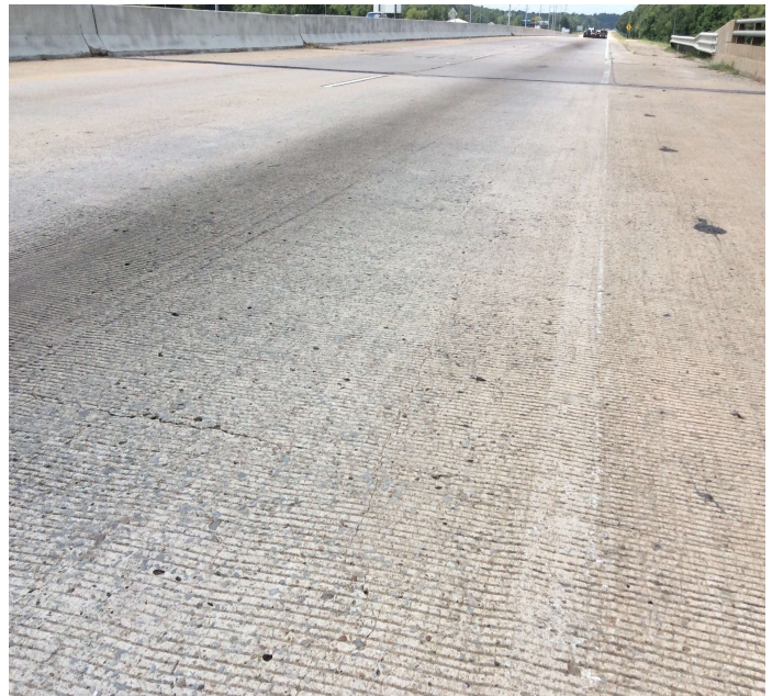
PHOTO 2 Description Span 1 Left lane Sealable map cracking.
