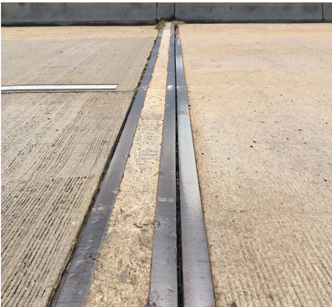
PHOTO 1 Description Bent 2 expansion joint deteriorated.
