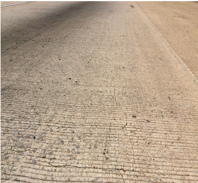
PHOTO 1 Description Deck cracking typical
